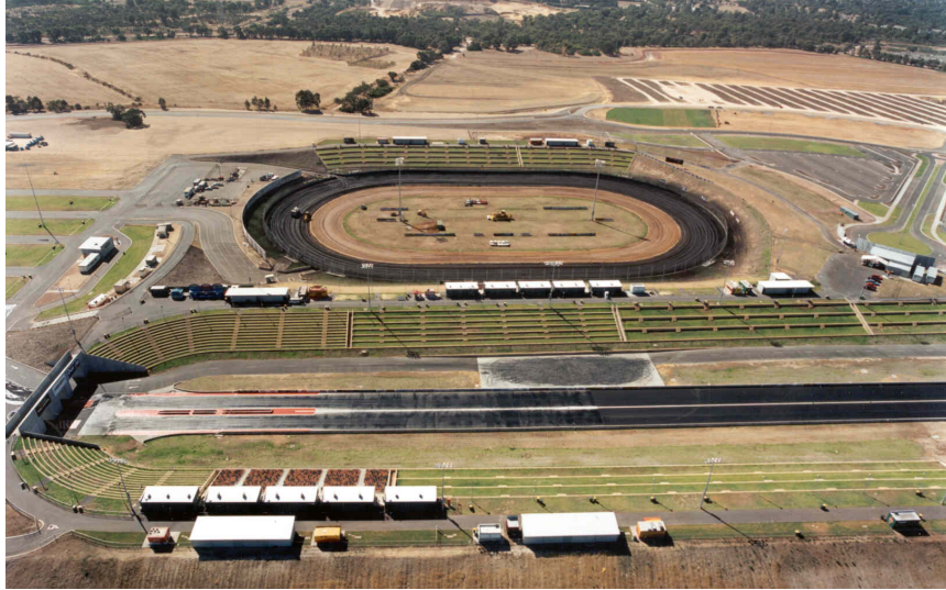
Motor Sports Complex built partially over the original residue storage areas.
