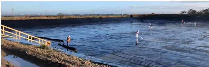
Above: Detailed pressure washing of the centre pond liner.
