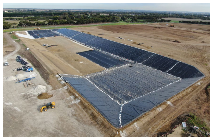
Above: Composite liner installation.
