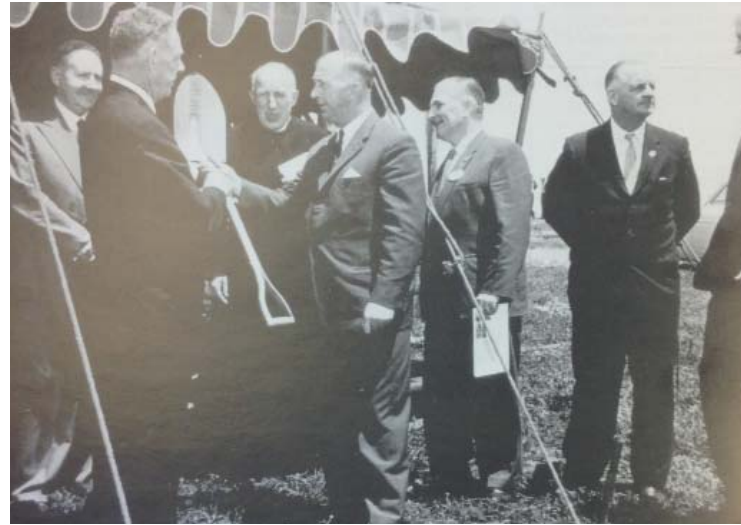
Breaking ground for the smelter in 1961. Image from White Gold, Geoffrey Blainey.
