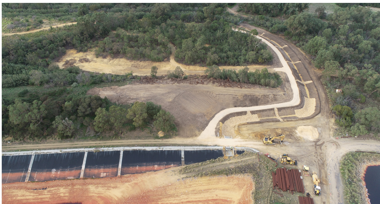
Figure 8-2: Cooling Pond Spillway
