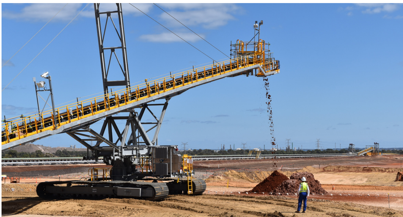
Figure 8-3: Bauxite Residue Filtration Bypass Emergency Stacker
