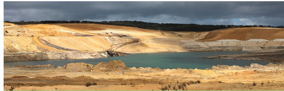
SOUTH WALL REPROFILING WORKS
