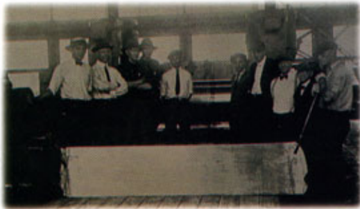
The First Slab
