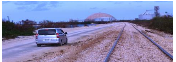
After: The railway line back in place and the road cleared.
