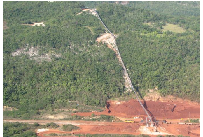
The RopeCon System takes bauxite from the South Manchester Plateau to the railhead at St. Jago.
