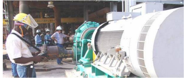
Technician carrying out vibration checks on pumps and motors during commissioning.
