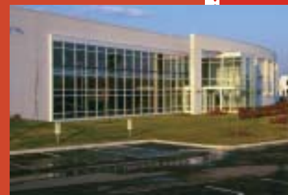
The Laval Casting facility
