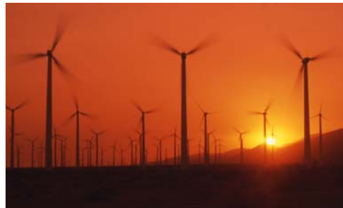
Photo courtesy of 3 Phases Energy
