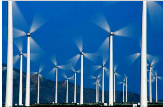
Photo courtesy of 3 Phases Energy
