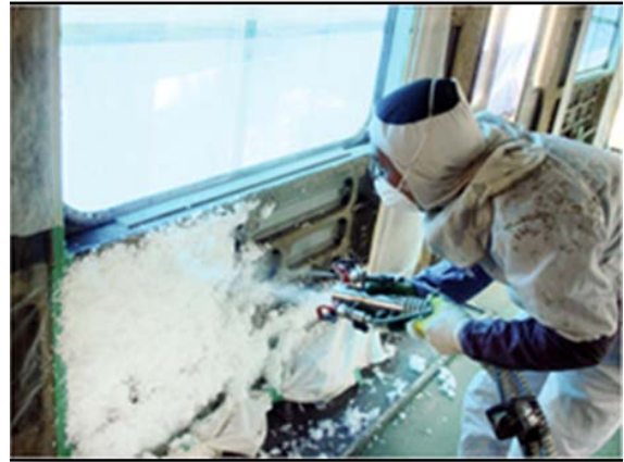
FIGURE 5 – Worker spray-coating aluminum structure with fire insulation.
