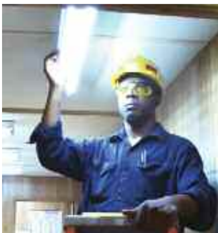
● Employee of Jamalco installs LED lamp: illumination costs are reduced by 33%
