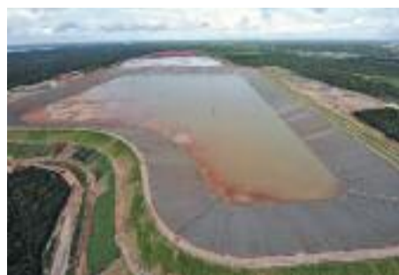
● Aerial view of the Bauxite 5 Residue Area
