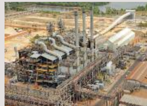
③ Calcining: In this stage, calciners 3 and 4 eliminate the molecular water contained in the hydrate, so that only aluminum oxide (alumina) will be produced, either for exports or for processing into metallic aluminum by smelting.
