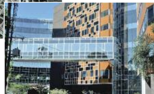
● Glasses glued with silicon or in frames for the three new buildings will use Alcoa's Cittá Due line window frames.
