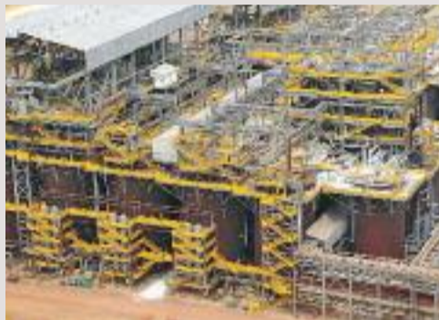
② Precipitation: In this process, the alumina contained in the green liquor (extracted from Digestion) as an aluminate, precipitates as a hydrate. This happens because of the decrease in temperature and pressure. Precipitators will supply the Refinery with the holding time and volume required to absorb the increase of flow in the Digestion units.
