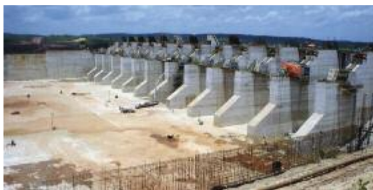
● Spillway of the Estreito Plant that conducts water from the Tocantins River
