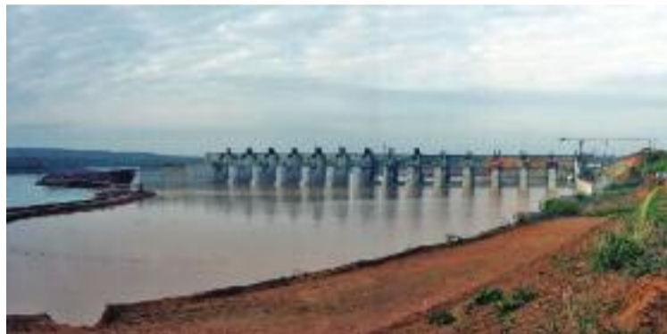
● Spillway of the Estreito Plant that conducts water from the Tocantins River
