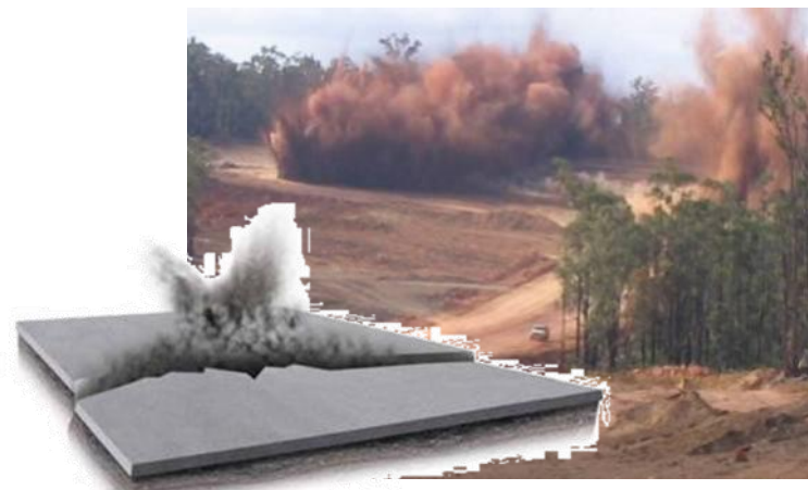
After Secondary Overburden Removal this hard, undulating surface caprock layer is exposed and ready to be broken up
