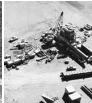
Erection of No. 1 original crusher at Huntly, 14th August 1975
