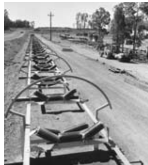
Tail end of Del Park Conveyor, 20th January 1975
