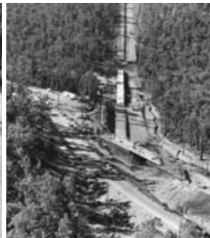
Del Park Road bridge and Conveyor bridge construction, 14th August 1975
