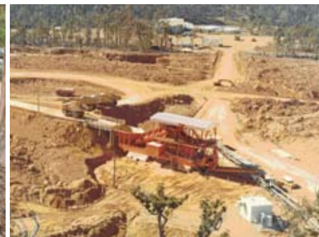
The first crusher on site at Huntly mine, 1976
