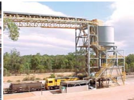
450 HOK Train Loading Station at Pinjarra refinery
