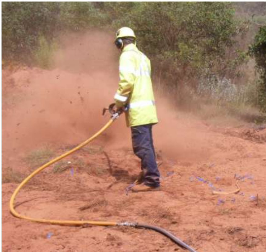
Figure 2: Displacement of the top 250 mm of sand to expose the surface root-plate using the Air-spade ® .
