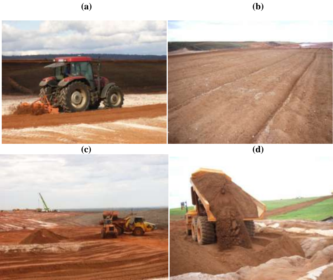
Figure 28. (a) Mixing gypsum with residue sand by disc harrowing, (b) final product containing 1% gypsum, (c) gypsum-amended residue sand was stockpiled then loaded into haul truck, and transported sand to lysimeter, and (d) final load of gypsum-amended residue sand to lysimeter
