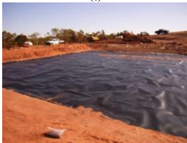
Figure 25. (a) Prior to commencing 2 nd lift, the PVC liner and protective HDPE liner were folded flat across the lysimeter surface, (b) an additional layer of HDPE liner was placed across the lysimeter surface to protect the liner, and (c) final protective layer before commencing 2 nd 1.5 m lift
