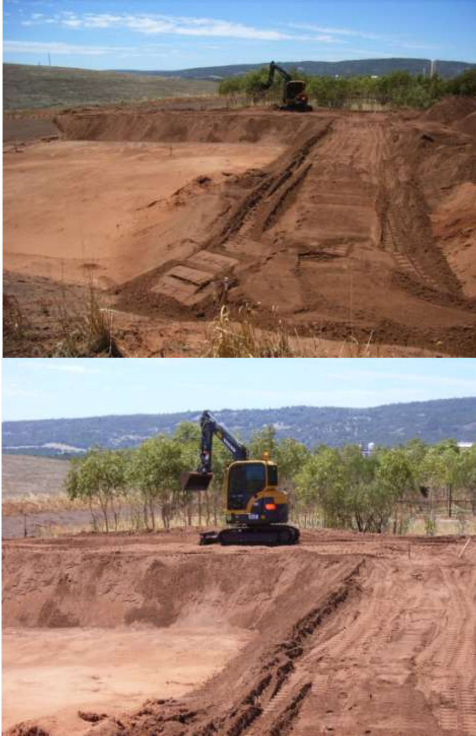
Figure 14. Construction of benches 1.5 m in height along eastern and southern boundaries
