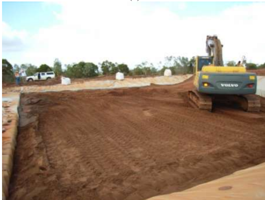
Figure 23. (a) Commencing to fill the lysimeter (1.5 – 3 m depth) with unamended residue sand, and (b) completion of filling the 1.5 – 3 m depth interval with unamended residue sand
