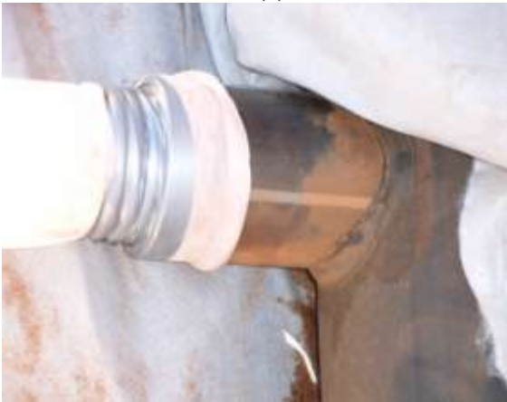
Figure 22. (a) Replacing filter sock on draincoil, (b) draincoil attached to sump drain pipe, (c) sealing draincoil to sump drain connector, and (d) installed draincoil at 2.5 m spacings
