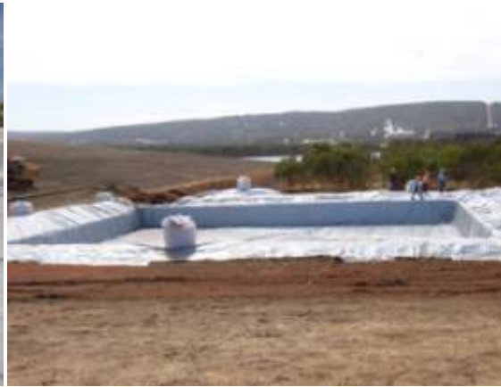
Figure 19. (a) Preparing liner for installation, (b) about half way through liner installation, (c) liner fully installed, and (d) preparing to remove large creases in PVC liner
