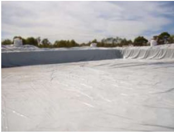
Figure 19. (a) Preparing liner for installation, (b) about half way through liner installation, (c) liner fully installed, and (d) preparing to remove large creases in PVC liner
