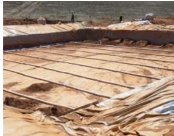
Figure 22. (a) Replacing filter sock on draincoil, (b) draincoil attached to sump drain pipe, (c) sealing draincoil to sump drain connector, and (d) installed draincoil at 2.5 m spacings
