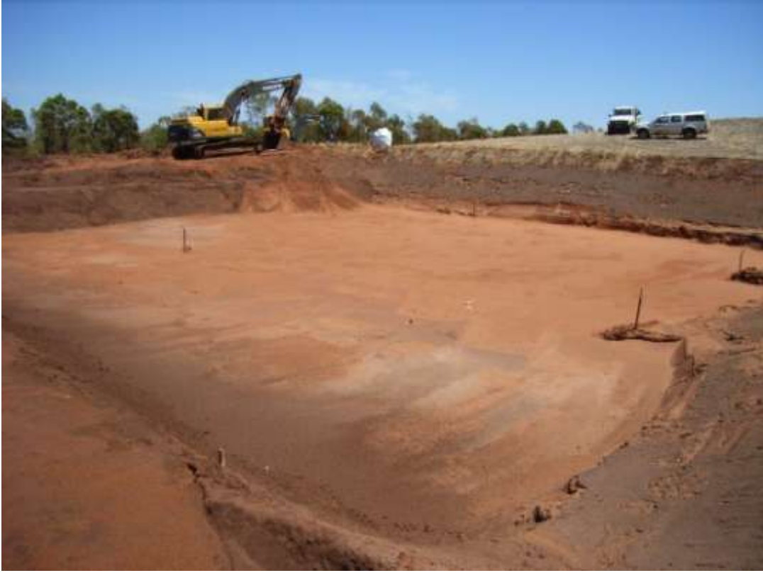
Figure 11. Base of new lysimeter after removal of 0.2 m of residue sand and vegetation
