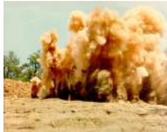
Blasting and ripping
