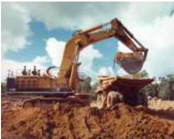
Load bauxite into haul truck
