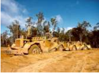
Scrape off Topsoil
