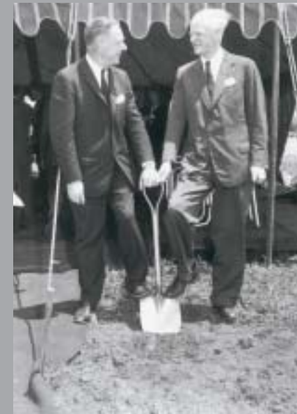
above – J.C. Smith and Sir Lindsay Clark 'breaking the ground' for the Point Henry smelter, 1961.
