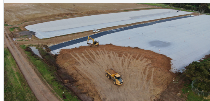
Capping subsoil placement | Moolap landfill site cell five
