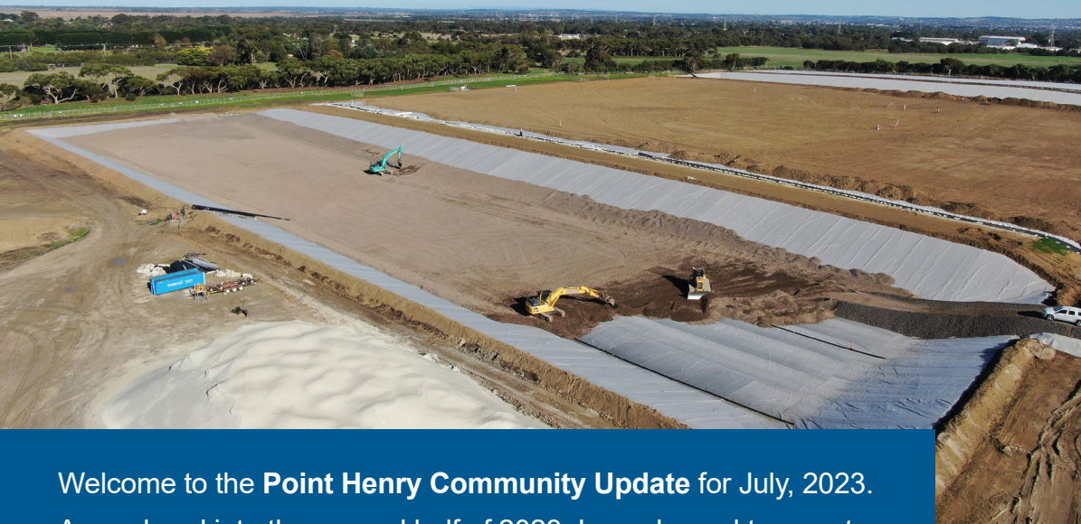
Leachate aggregate placement | Moolap landfill site cell seven
